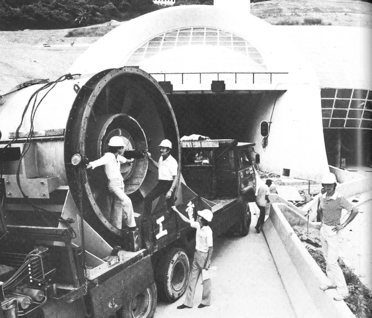
Ventilation fan for the Aberdeen Tunnel
